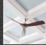
CEILING OIL BOUND DISTEMPER
