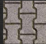
INTERNAL ROADS INTERLOCKING BLOCKS/ TREMIX CONCRETE ROAD
