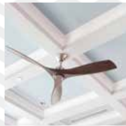
CEILING OIL BOUND DISTEMPER
