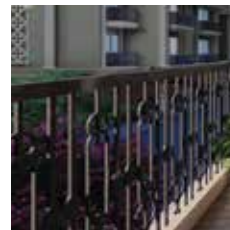
RAILING WROUGHT IRON RAILING
