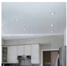
WALL / CEILING OIL BOUND DISTEMPER
